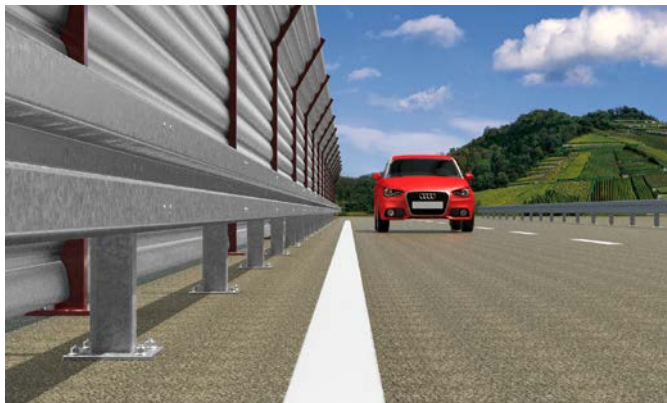
Sound insulation walls
