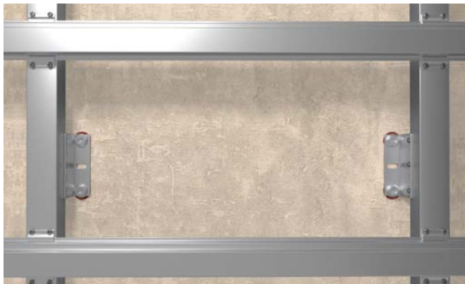
Façade substructure
